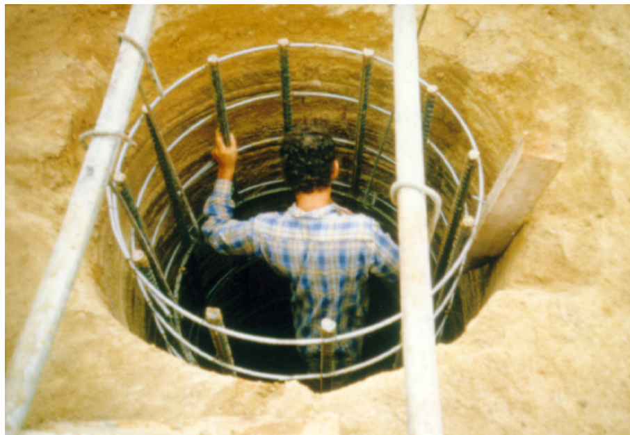
Figure 6.2: Preparations for pouring the siderostat foundations at SUSI.
