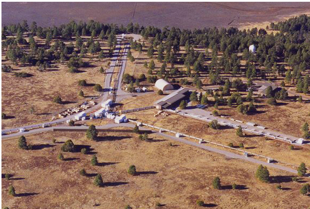
Figure 10.1: An aerial view of the NPOI showing the array as viewed from the north-east. The road surrounding the array can be seen along with parts of the north (right) west (center) and east (left) arms of the imaging array (station piers and vacuum feed lines visible). The astrometric siderostat shelters are the white structures at the array center. The beam-combining laboratory is the long structure to the right of the array center, with the ‘long’ delay line vacuum tanks (under construction) extending towards the north. The interferometer control building appears at the far right-center.
